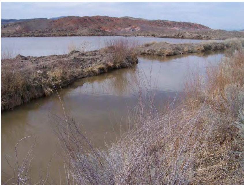
Figure 10. Gunnison Detention Pond (water is diverted from the canal to the pond shown in the background and then flows back into the canal).
