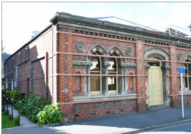
URM retrofitted building - 2011 Mw 6.1 Christchurch, New Zealand earthquake. Photo: EERI/Fred Turner.
