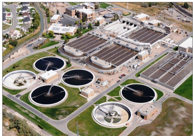
Wastewater treatment plant located in Salt Lake County. Photo courtesy of South Valley Water Reclamation
