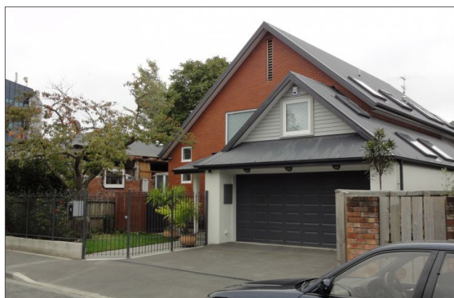
Engineered residential home with extensive foundation with piles. Other homes around the neighborhood suffered significant damage due to liquefaction - 2011 Mw 6.1 Christchurch, New Zealand earthquake. Photo: EERI/Justin Marshall.
