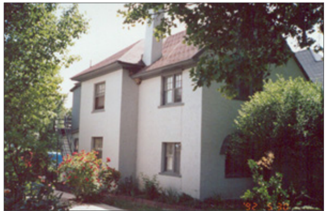
Example two-story URM residence. Photo courtesy of Barry Welliver.
