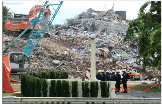
Debris from the catastrophic collapse of the Pyne Gould Corporation - 2011 M_w 6.1 Christchurch, New Zealand earthquake. Photo: EERI/Troy Morgan.
