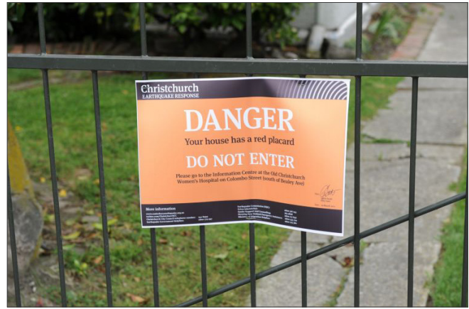
Notice to resident of red tagged house - 2011 Mw 6.1 Christchurch, New Zealand earthquake. Photo: EERI/David Swanson.
