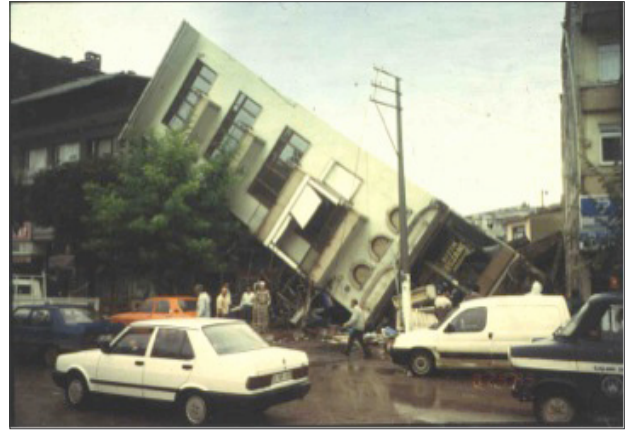
Figure 17. Building in Adapazari, Turkey that tipped over due loss of bearing capacity during the 1999 Kocaeli, Turkey earthquake. Photo by T.L. Youd.
