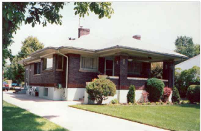
Example one-story URM residence. Photo courtesy of Barry Welliver.
