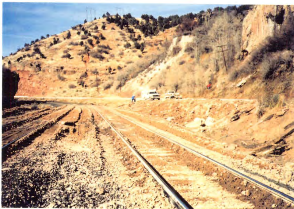
Area of Railroad tracks covered by the toe of the slide (After cleanup)
