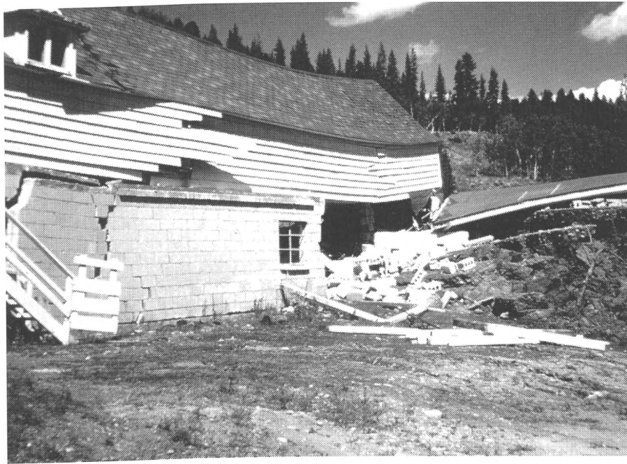
Figure 3. Barn that crossed the Red Canyon fault and was offset during the 1959 Hebgen Lake, Montana, earthquake. The back wall of the barn is crushed and the whole structure is disrupted. (Photograph by K. Steinbrugge)
