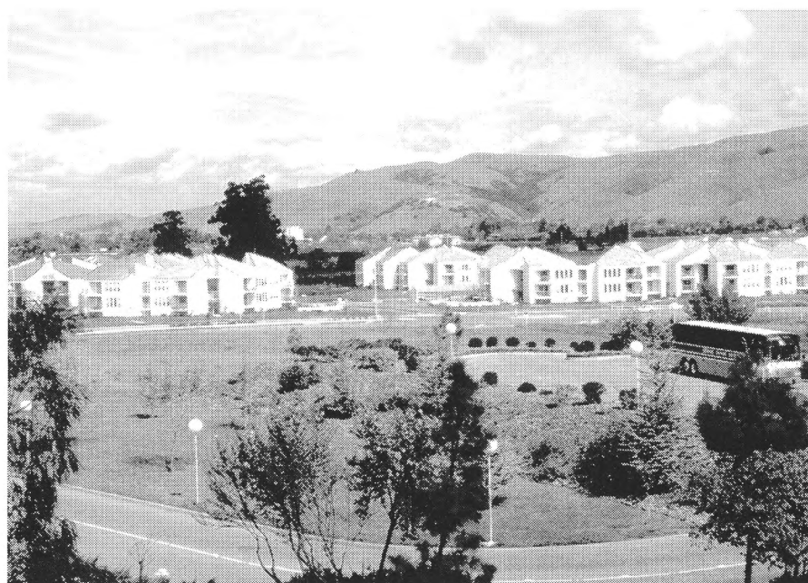
Figure 4. Example of avoidance mitigation of surface-faulting hazard along the Hayward fault in California. A major trace of the fault passes from the right of the bus through the gap in the apartment buildings. This gap is the set-back area to avoid the fault; the area was replanned to be a small, open, grassy area and parking spaces. Many communities in the Basin and Range Province have the opportunity to guide planning such that buildings and other structures avoid crossing faults when it is unnecessary. (Photograph by C. dePolo)
