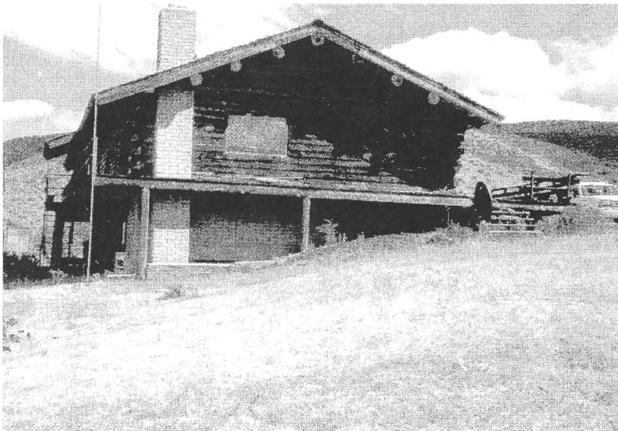
Figure 2. House built across fault scarp in a rural Basin and Range Province setting. There is little developmental pressure here and the house could have easily been offset from the fault had the owner known it was an active fault. (Photograph by C. Willoughby)
