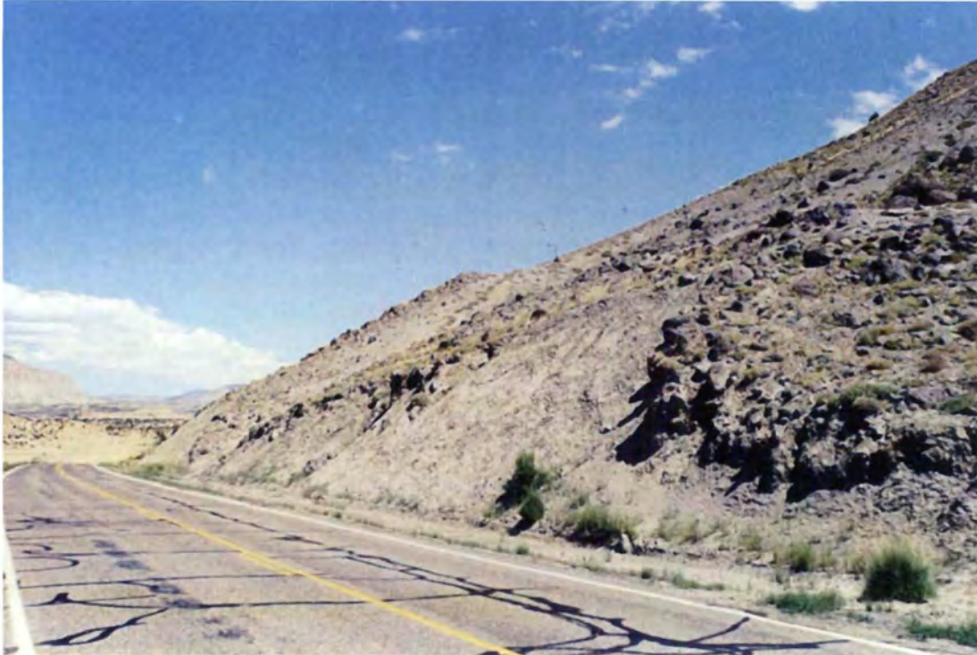
Figure 3. C-rated slope near Emery, Utah.
