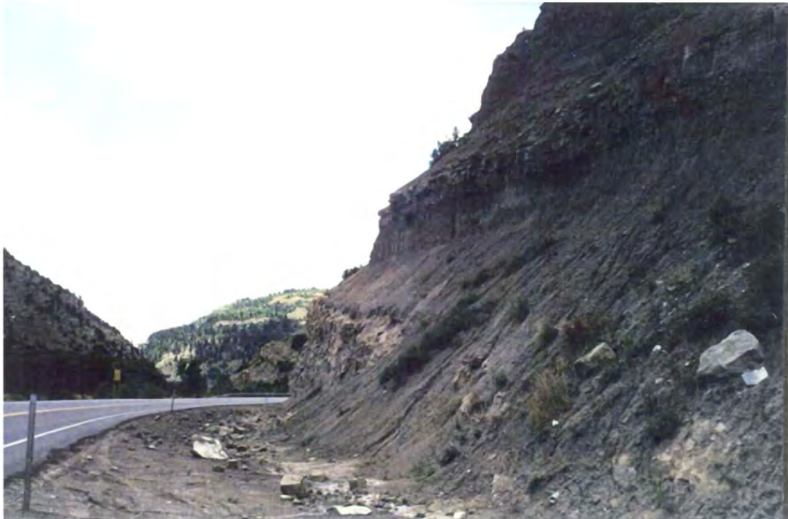
Figure 5. B-rated slope near Colton, Utah.
